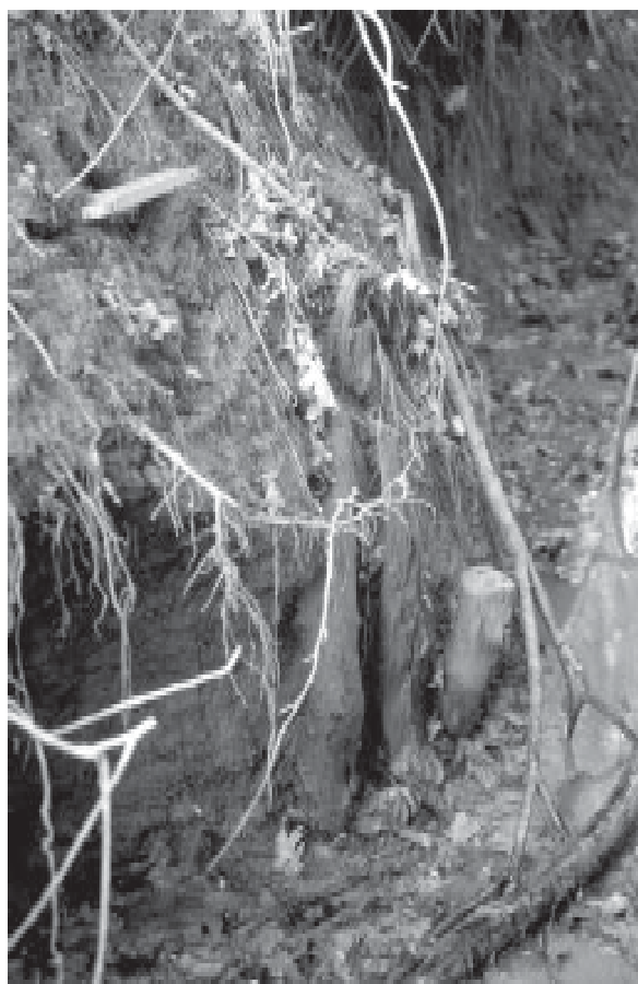
Sl. 2: Jarek Hočevarica. Fig. 2: The Hočevarica ditch.
